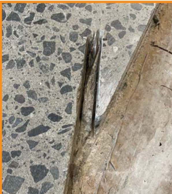
Installation of PNSX™ at Home of the Arts, Gold Coast to repair damage to new polished concrete floor during construction.
