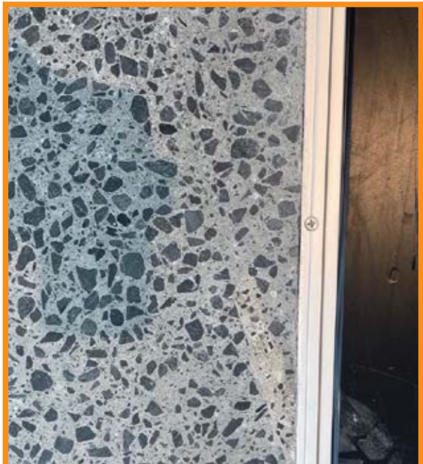
Installation of PNSX™ at Home of the Arts, Gold Coast to repair damage to new polished concrete floor during construction.
